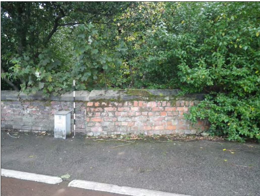
Plate 16: Detail shot of the reworked western entrance (1m scale)
