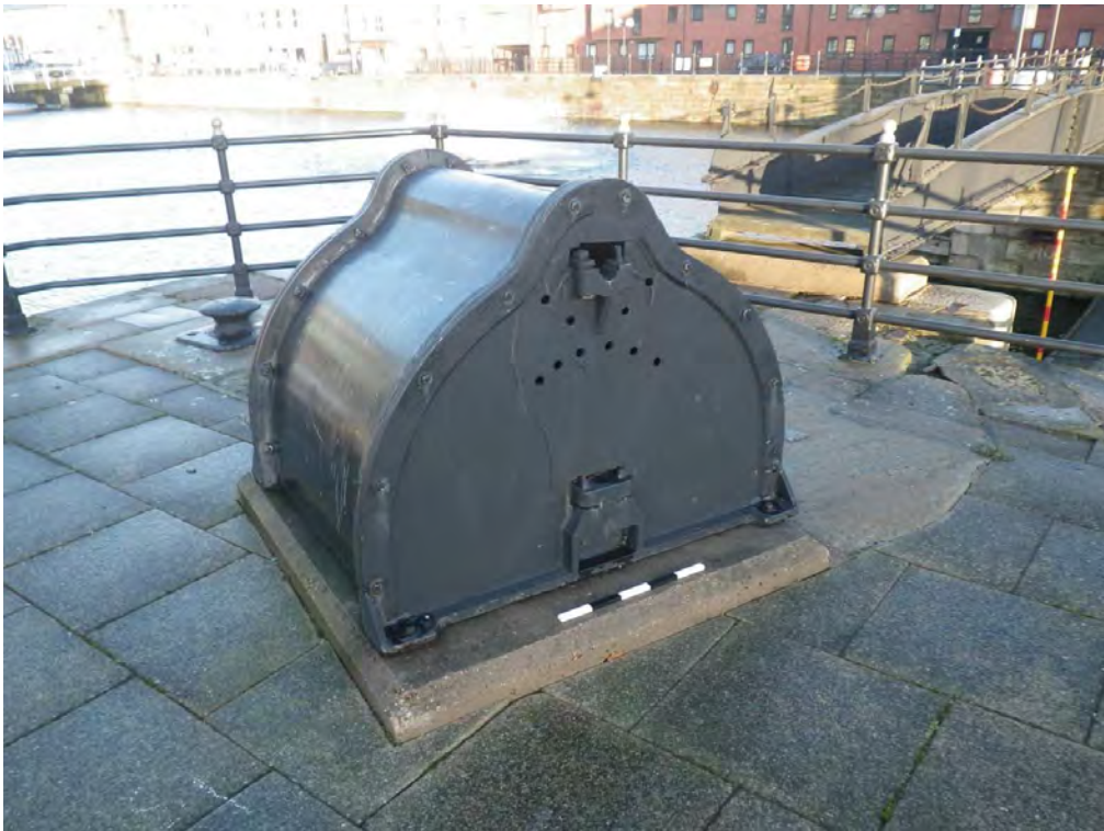
Plate 7: Winch base (item 18, same as items 19, 20 and 21), looking north-east
