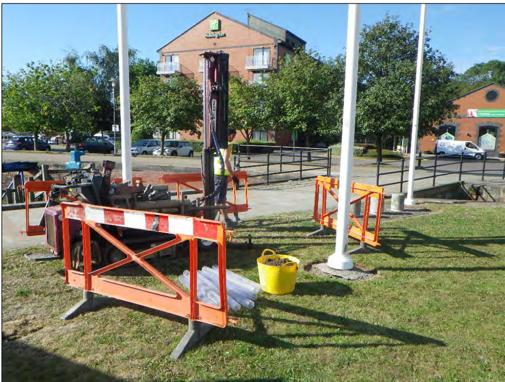
Plate 2: Window sample (WS16) extracted north of Humber Dock
