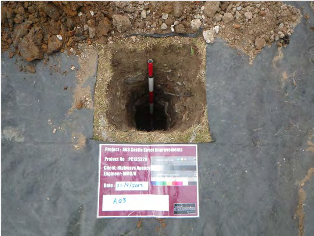
Plate 45: Test pit A03, prior to Static Cone Penetration Testing, looking north (1.2m scale)
