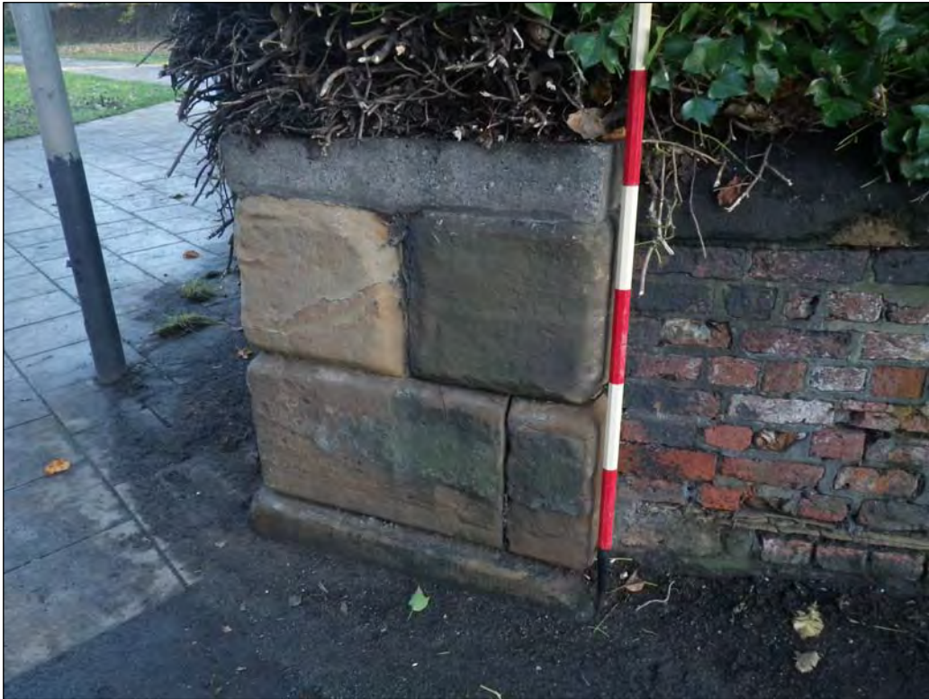
Plate 17: Stone gate pier exposed at north end of western gaol-yard wall after later clearance of vegetation, with northern wall of burial ground abutting its eastern side
