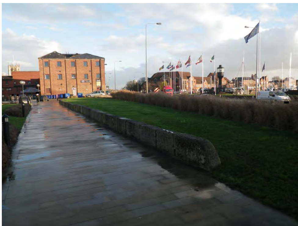
Plate 4: Low retaining wall (item 13), looking east
