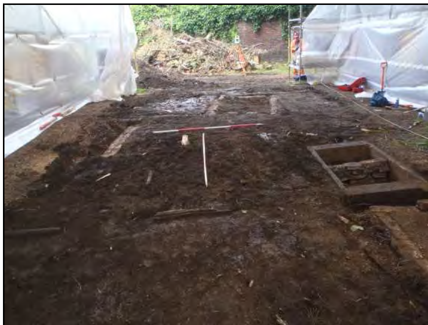
Plate 12: Trench B with the various red brick-built tombs exposed at or just below ground level, and the sandstone box support for ledger 1179 visible to the centre right. Viewed facing east
