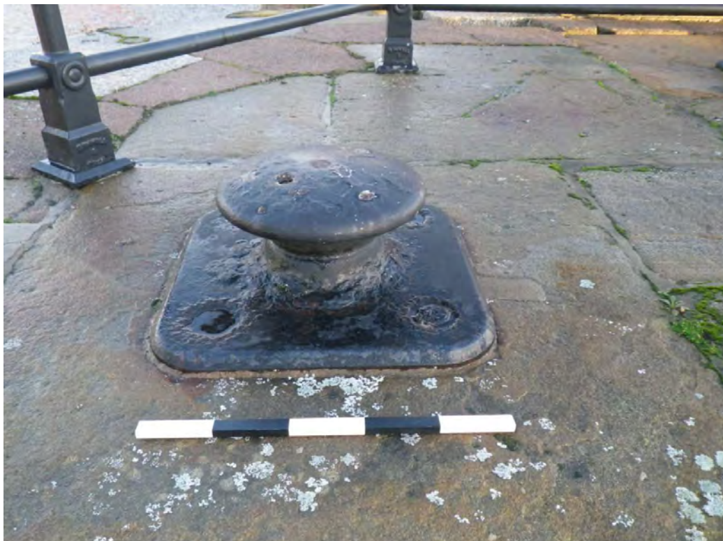
Plate 6: Cable guide (item 17), looking east
