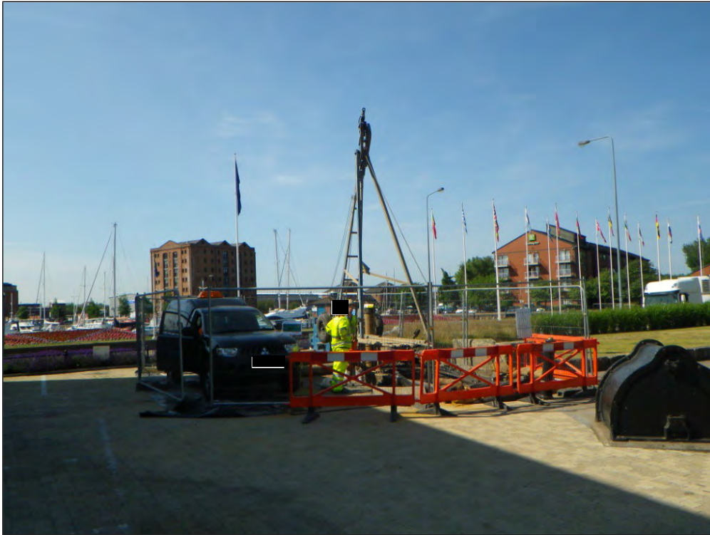
Plate 1: A working shelling augur rig in self-contained compound, drilling BH39
