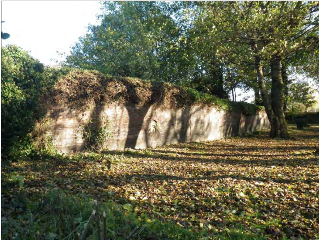
Plate 23: The western face of the gaol-yard wall exposed following removal of some vegetation
