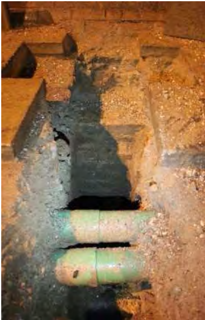
Plate 6: Wall in southern end of the part of Trench S5 that was excavated through the pavement
