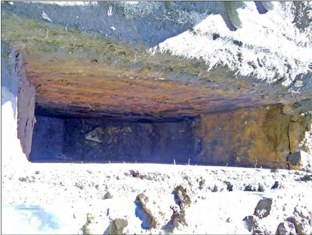
Plate 51: TP18A showing stone foundation (G), looking south
