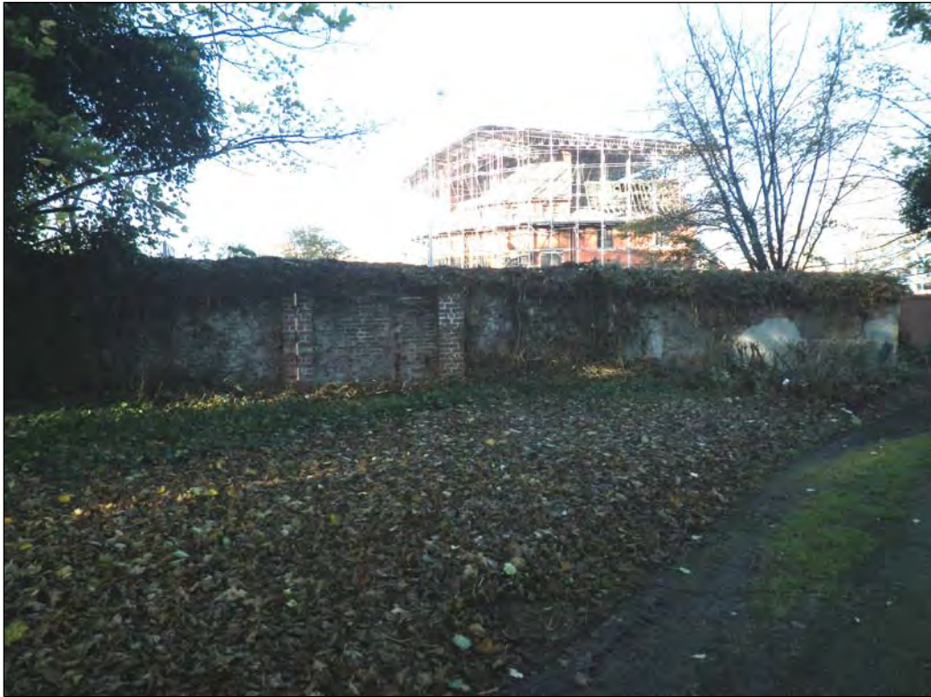
Plate 27: Eastern part of the gaol-yard wall southern face following removal of vegetation
