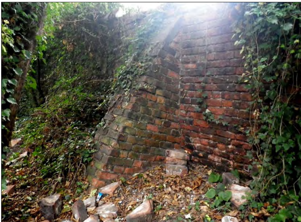
Plate 12: Detail shot of the west-wall buttress; note disturbed coping bricks on ground
