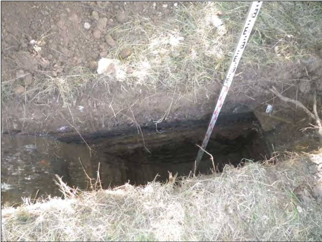
Plate 47: TP04 fully excavated, looking west
