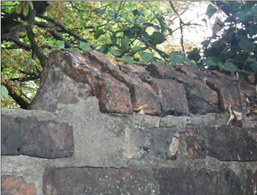
Plate 7: Detail shot of the original coping to the west wall
