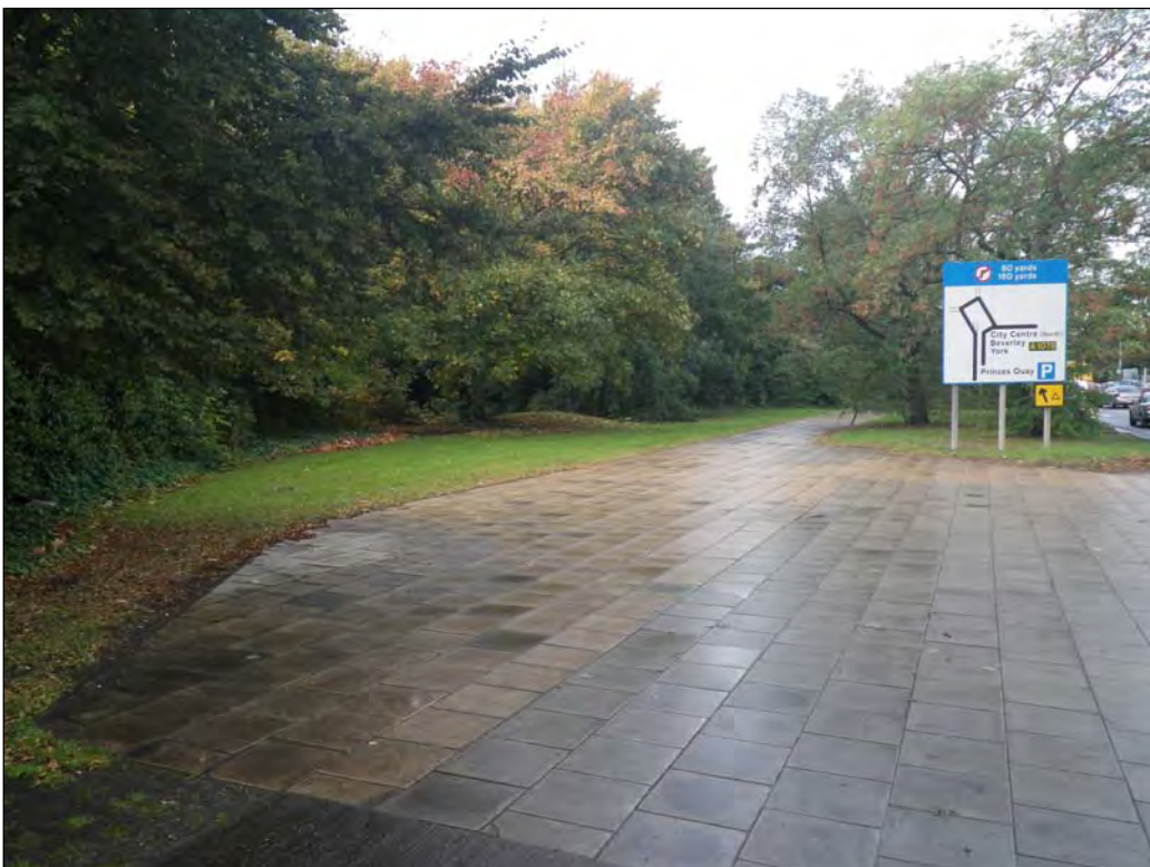
Plate 18: The site of the former gaol on Castle Street viewed from the east. The former gaol-yard walls and walls of the burial ground are almost entirely obscured by vegetation
